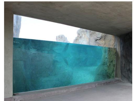
R-Cast® panels are an ideal choice for multiple types of exhibits. In this example, the acrylic is thick enough to withstand the force of a polar bear, yet completely transparent, allowing for views of the outside.
