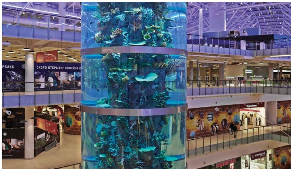
The aquarium at the Avia Park shopping center in Moscow is 75 feet tall. The tank is constructed of seven sections of R-Cast® acrylic, which weigh up to 26,000 pounds each. The acrylic is up to eight inches thick to retain the 98,000 gallons of water within the tank.
